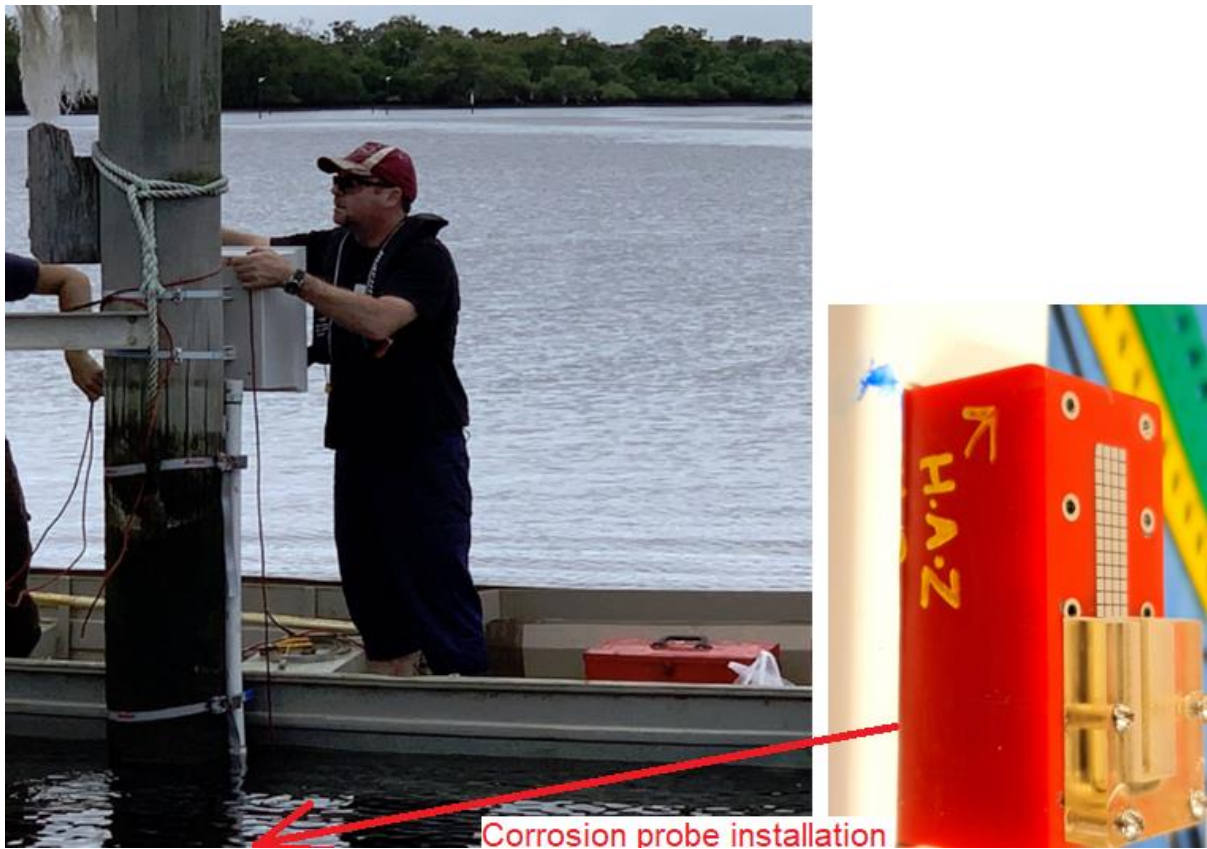
Figure 3. Field test locations and field testing setup and measurements at Taylor's Beach NSW field testing site for acquiring localised corrosion data.
